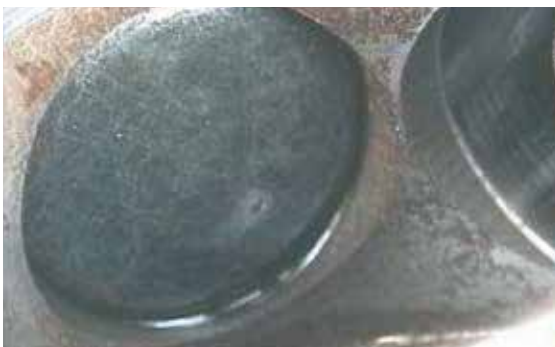
Corrosion at the high-pressure pump housing
