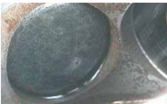
Corrosion at the high-pressure pump housing
