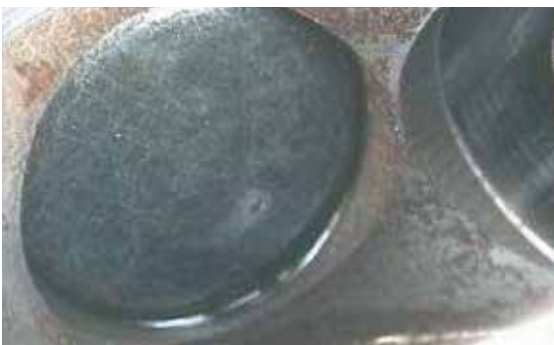
Corrosion at the high-pressure pump housing
